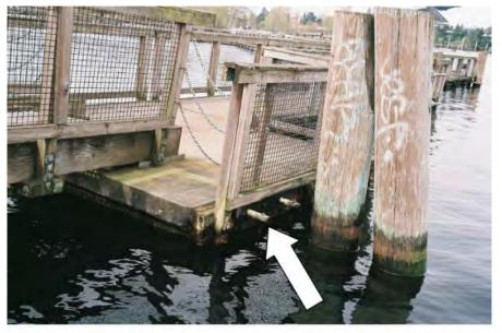
**PHOTO No. 7:** Walkway, Float Anchor Piles No. 16 and 16 Batter - Note the float anchor hoop is not aligned with the piles and has been cut off. Also note the pontoons are floating unevenly due to the weight of the interconnecting ramp.
